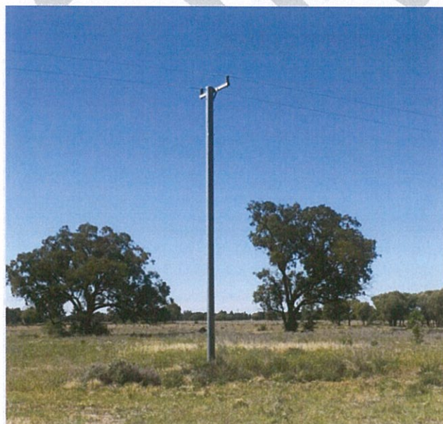
Photograph 3: Overhead powerline situated on the subject site
